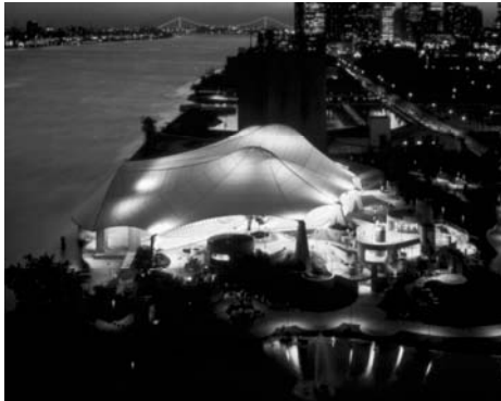
Figure 1-11 Chene Park Amphitheater, Detroit, Michigan, 1990 (Photograph courtesy of Birdair, Inc.)
