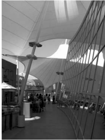
Figure 3-3 Premium Outlets Mall, Las Vegas NV PVC-coated polyester fabric (Photo courtesy of Fabritec Structures)
