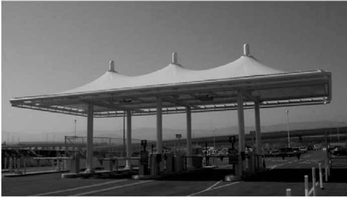
Figure 8-4. San Francisco International Airport Parking Canopy (Photograph with permission from Craig G. Huntington)
