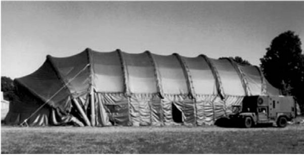
Figure 3-5 Department of Defense TME system High pressure inflatable air beams in Kevlar tubes with PVC coating
