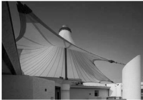
Figure 3-7 Pensacola Municipal Pool, FL Silicone coated glass fabric
